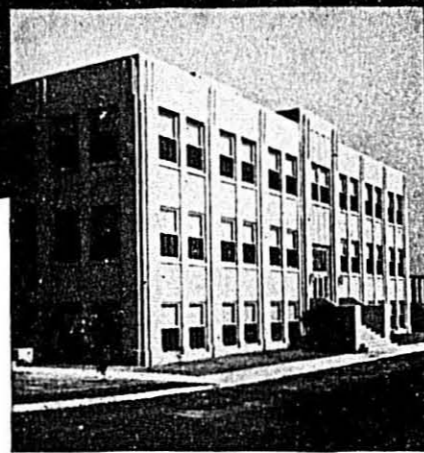
The Staley Chemical Research Building at Staley's main plant.
